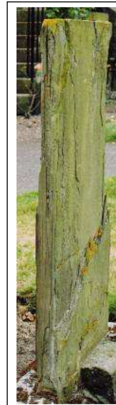
Figure 76 Major contour scaling on carved surface
