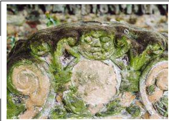
Figure 76 Major contour scaling on carved surface
