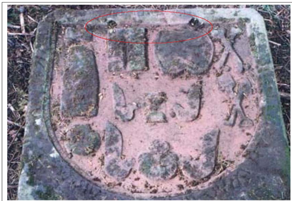
Detail showing drainage holes
