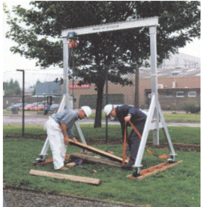
*Illustration 2. Preparing to lift a stone – securing the stone to a wooden batten.*
